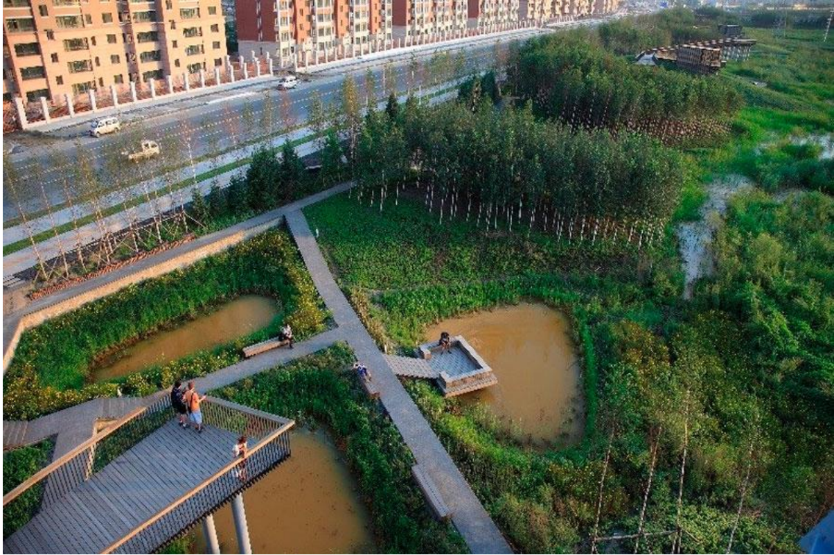
Urban storm water park in the city of Harbin in China provides multiple ecosystems services: collecting cleansing and storing storm water which then infiltrates it into the aquifers. In addition to recreating natural habitats it provides a great public space for recreational use.
